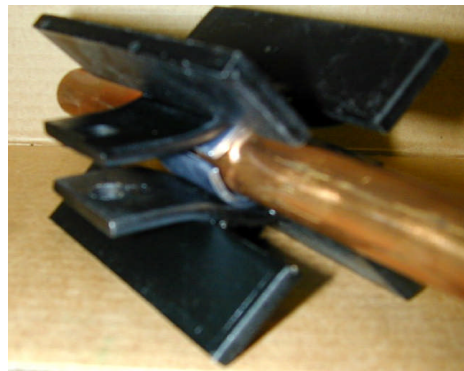
4. Attach upper half of spider clamp as shown
