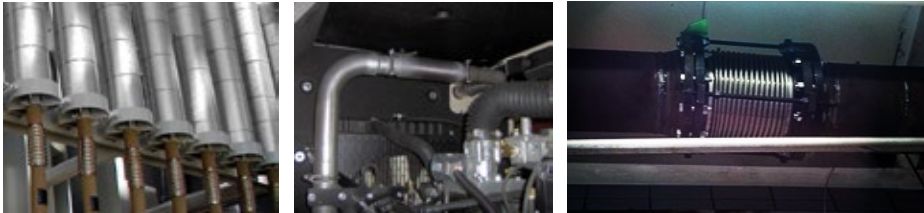
Lined Metal Expansion Joint
