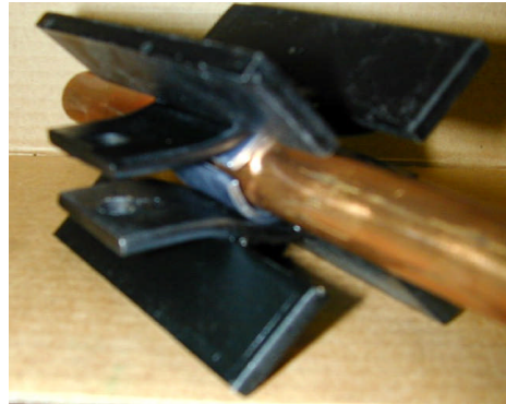
4. Attach upper half of spider clamp as shown
